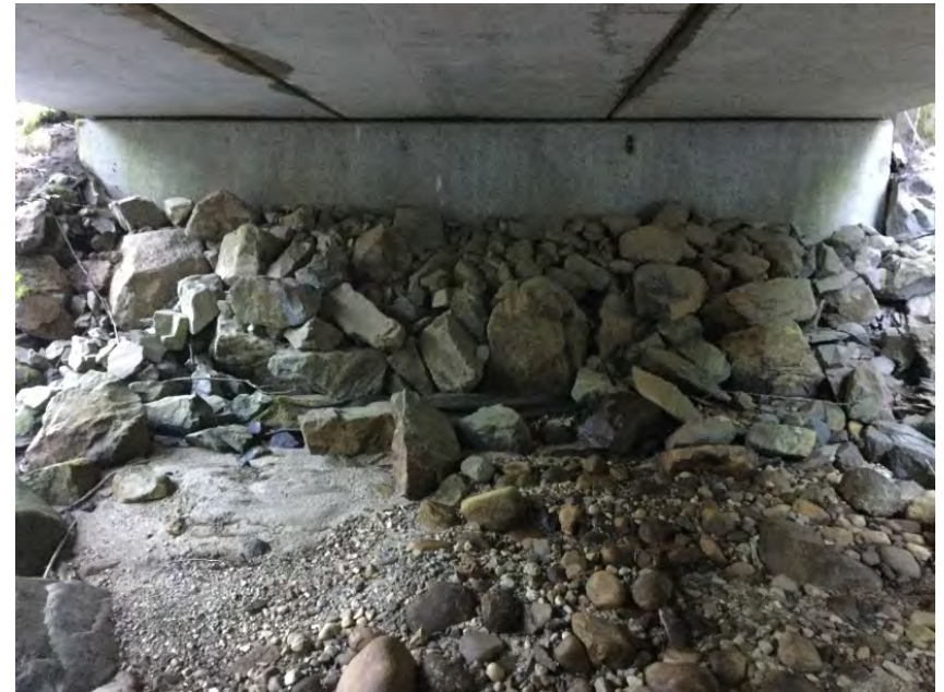
Right Bank Abutment when facing downstream
