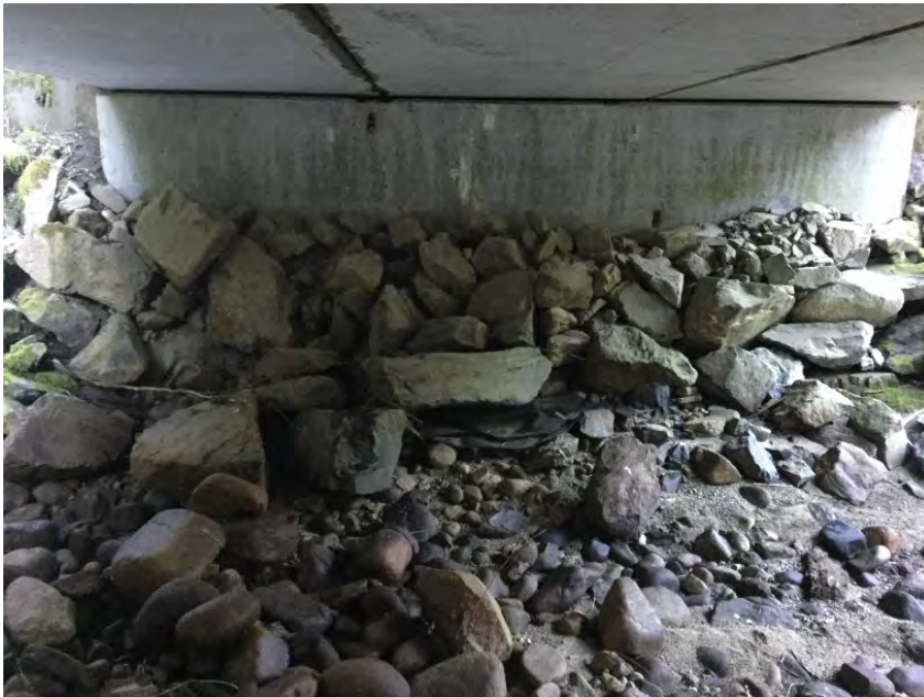
Left Bank Abutment when facing downstream
